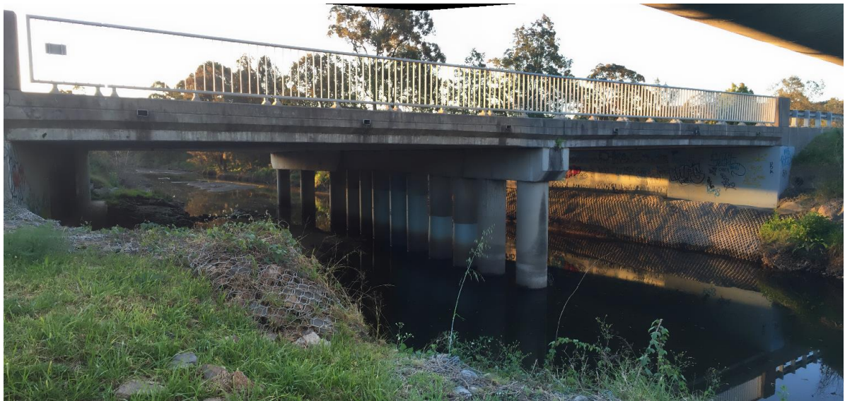
Figure 2-2 Lake Road Bridge over Winding Creek, Glendale
